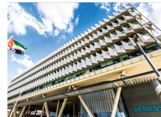
Siemens Energy Middle East HQ
